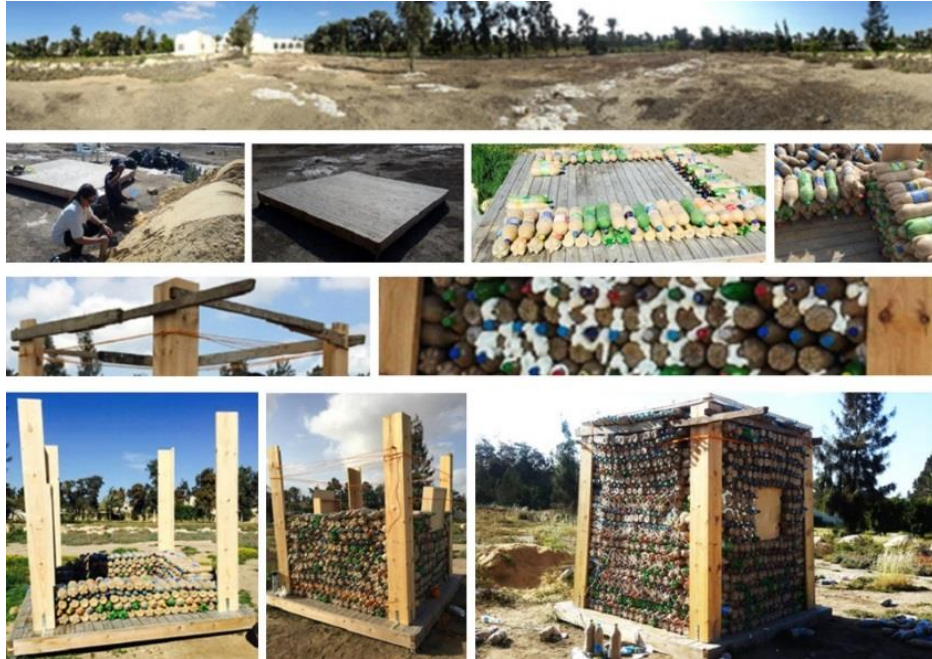
Fig 1: Bottle walls building Process
