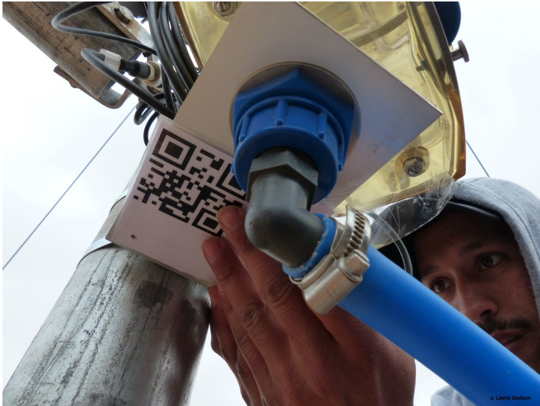
Figure 2. The water manager uses a tablet computer and QR codes to monitor the fog harvesting infrastructure. Photo by Leslie Dodson.
