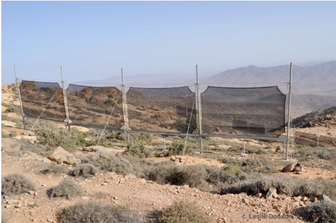
Figure 1. Dar Si Hmad's Phase 1 fogwater harvesting system includes 600 square meters of fog nets. Photo by Leslie Dodson.
