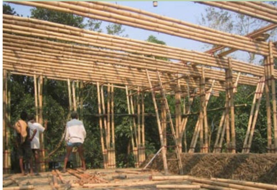
Placing the "Weller"-mix on the foundation by hand.
