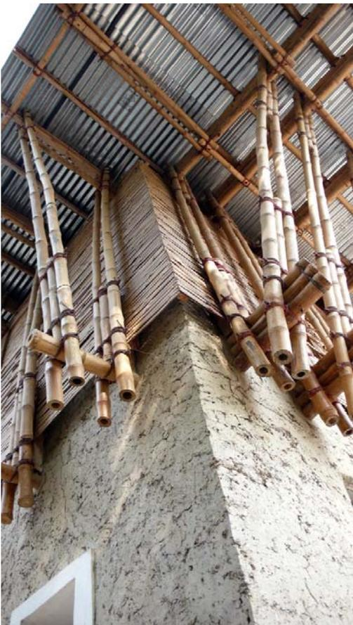
The roof is a frame construction consisting of beams - four layers of joined bamboo sticks- and vertical and diagonal poles..
