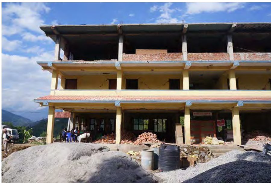
Reinforce concrete structure. (Note racking of center storey)
