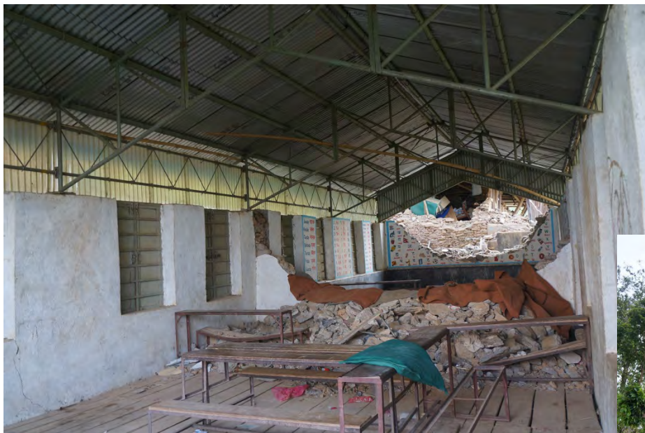
School built by Japanese consisting of metal framed structure. Note that the stacked stone end and divider walls have failed, but the metal columns and roof trusses are sound and are anchored to concrete footings.
