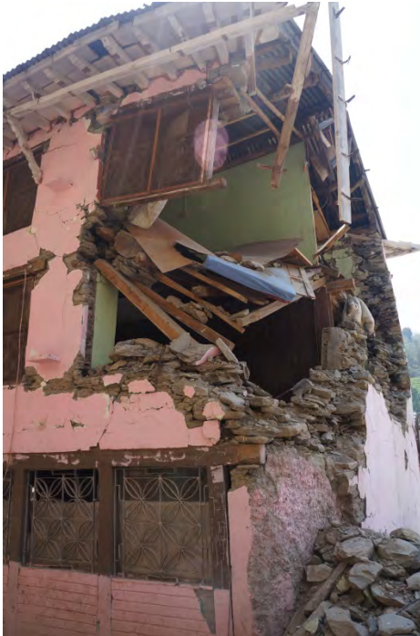
Stacked stone structure with wooden lintels on top of wall which steel roof trusses are anchored to.
