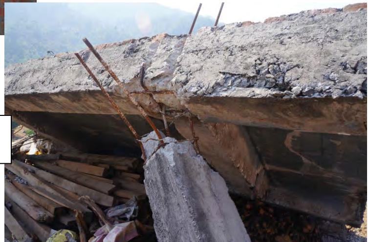
Column pulled out of beam due to lack of hooks
