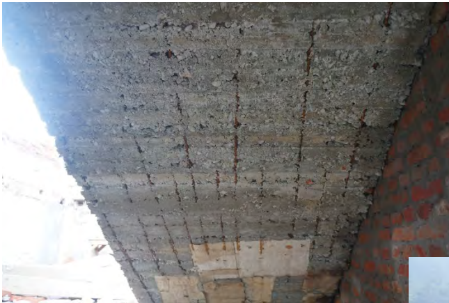
Rebar exposed at the bottom of a beam due to lack of support in forms during construction
