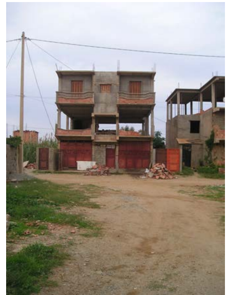
Figure 12: Typical building under construction
