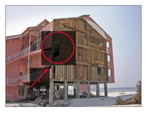
Several of the studs shown in Figure 11-19 were severely rotted, indicating long-term moisture intrusion behind the MEPS insulation. The residence shown in Figure 11-19 had a barrier EIFS design, rather than the newer drainable EIFS design (for another example of a barrier EIFS design, see Figure 11-21). EIFS should be designed with a drainage system that allows for dissipation of water leaks.
