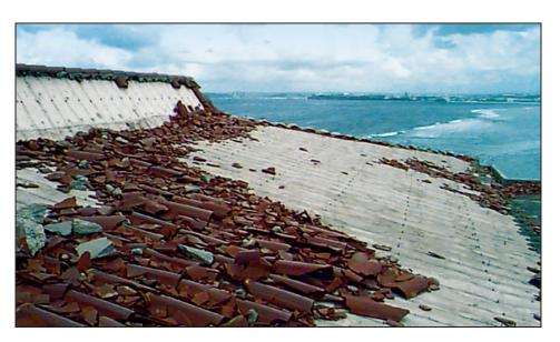
Figure 11-41. Blow-off of wire-tied tiles installed over a concrete deck. Typhoon Paka (Guam, 1997)
