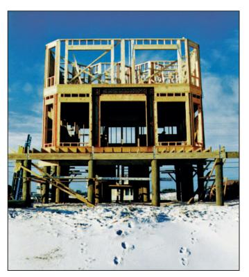
Figure 9-25. Steel moment frame with large opening
