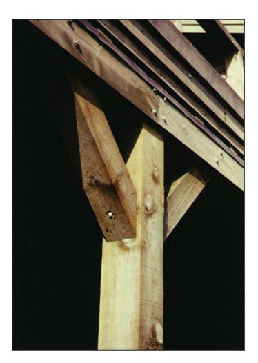
The feasibility of knee bracing is often governed by the ability to construct strong connections in the braces that connect the wood piles to the elevated structure.
