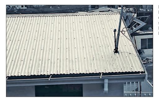
Figure 12-6. Damage caused by dropped overhead service, Hurricane Marilyn (U.S. Virgin Islands, 1995)
