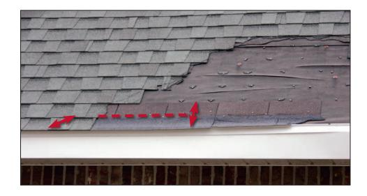
Storm damage investigations have shown that metal drip edges (edge flashings) with vertical flanges that are less than 2 inches typically do not initiate eave or rake damage. However, the longer the flange, the greater the potential for flange rotation and initiation of damage. If the vertical flange exceeds 2 inches, it is recommended that the drip edge be in compliance with ANSI/SPRI ES-1.
