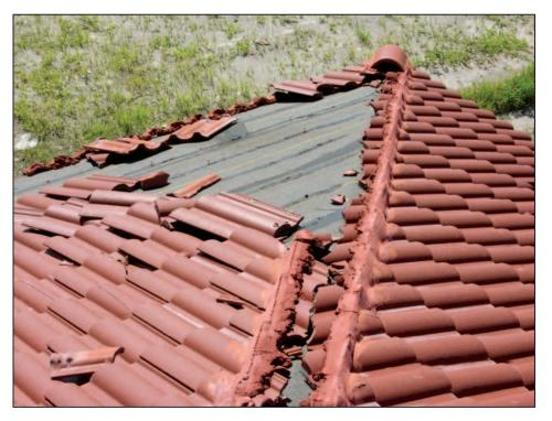
Figure 11-45. Blow-off of mechanically attached tiles. Estimated wind speed: 140 to 160 mph. Hurricane Charley (Florida, 2004)
