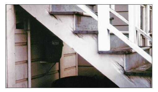
Using the alternative stair stringer installation shown in Figure 13-14 when the stair treads are either nailed onto a cleat or the stringer is routed out so the tread fits into the routed-out area. Even these alternatives allow water retention at end grain surfaces, and these surfaces should therefore be field-treated with wood preservative.
