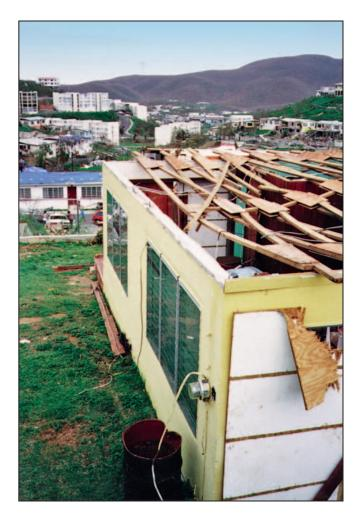
Figure 9-26. Gable-end failure caused by high winds, Hurricane Marilyn (U.S. Virgin Islands, 1995)
