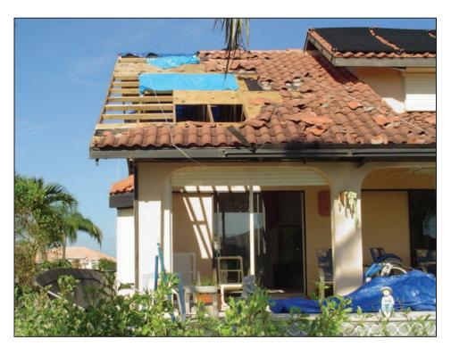
Figure 9-4. Load path failure in connections between roof decking and roof framing, Hurricane Charley (Punta Gorda, FL, 2004)
