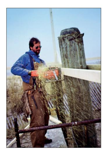
Figure 13-3. Improper overnotched wood pile SOURCE: PATTY MCDANIEL, USED WITH PERMISSION
