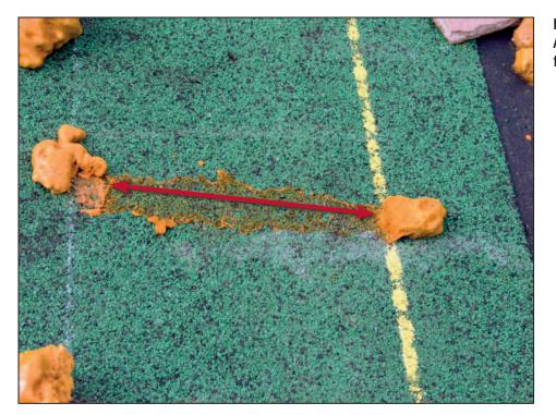
Figure 11-44. Adhesive that debonded from the cap sheet
