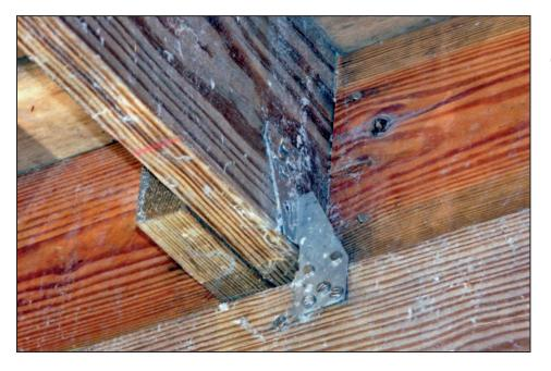
Figure 9-17. Metal joist-to-beam connector
