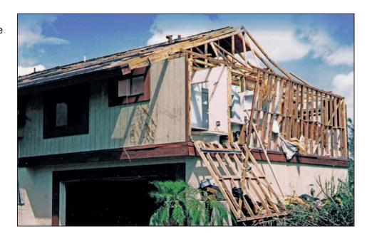
Figure 9-2. Load path failure in connection between home and its foundation, Hurricane Fran (North Carolina, 1996)
