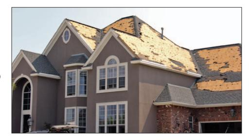
secondary protection requires an enhanced underlayment design. Design enhancements include increased blow-off resistance of the underlayment, increased resistance to water infiltration (primarily at penetrations), and increased resistance to extended weather exposure.
