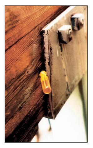
Figure 14-2. Wood decay behind a metal beam connector
