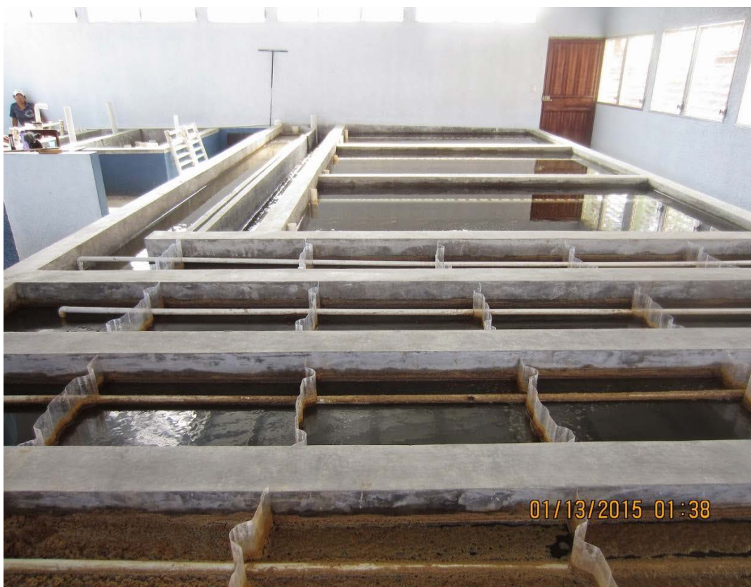
Figure 8. Interior view of the flocculator and sedimentation tanks at the Jesus de Otoro drinking water treatment facility.
