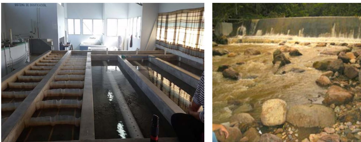
Figure 10. Left photo: Moroceli's flocculator (left) and three sedimentation tanks (right) with filtration in the background. Right photo: the water source is a small river that is very turbid after run-off events.
