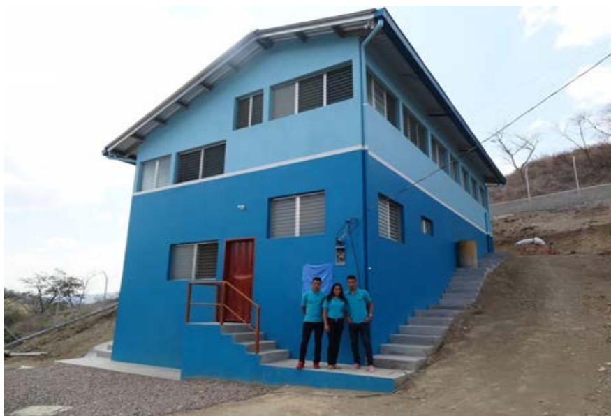
Figure 12. Exterior view of the AguaClara plant at San Matias. The compact layout of the water treatment plants makes it possible to enclose the entire facility inside a secure building.
