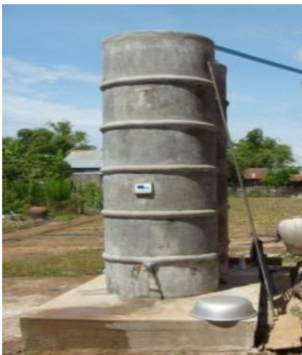
Figure 2. Concrete ring tank
