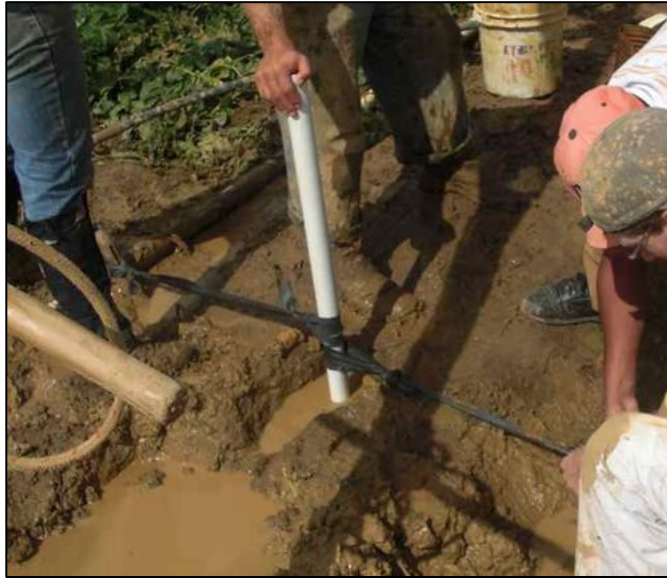
Figure 31 - Holding the casing in place with rubber strapping Image courtesy: Forsyth, Ramudu, Hindal, & Lazarus, 2010
