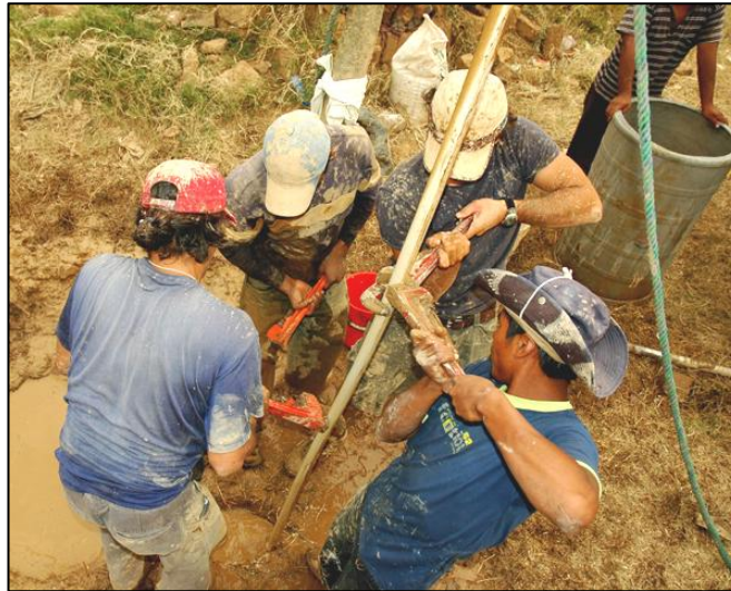
Figure 29 - Holding the drill stem with pipe wrenches
