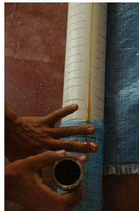
Figure 16 – Rice bags glued to filter
