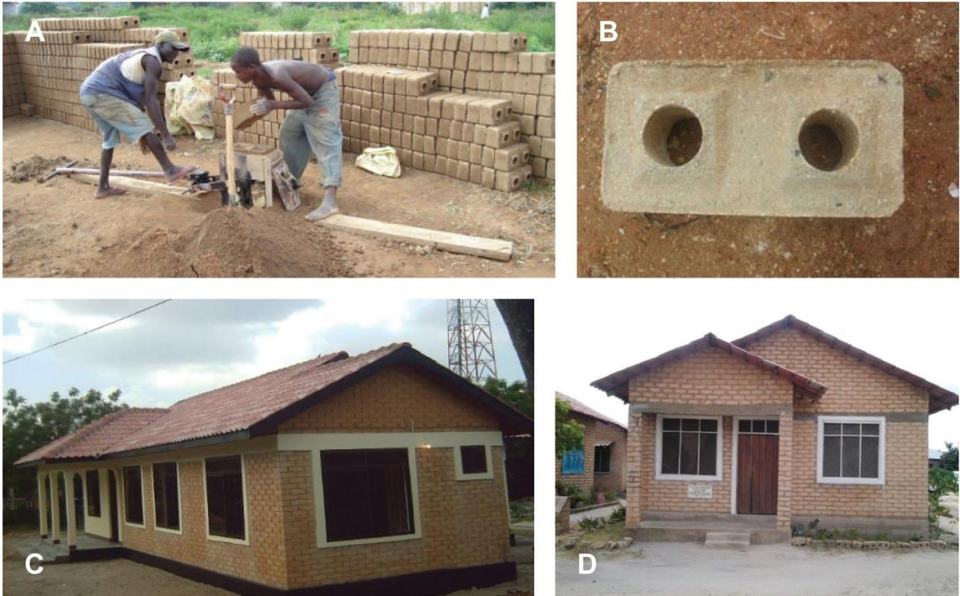
Figure 3. (A) Fabrication of interlocking soil-cement blocks; (B) Finished soil-cement block; (C) Construction made in 2000 by the NHBRA using interlocking soil-cement blocks in Tanzania; and (D) Example of a house built by the NHBRA in Chamazi, Dar es Salam. Source: NHBRA<sup>43</sup>
