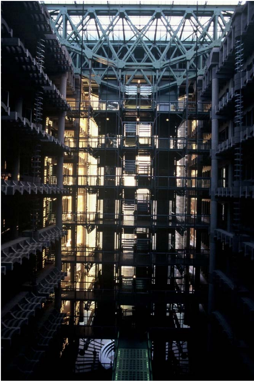
• Atrium looking west
