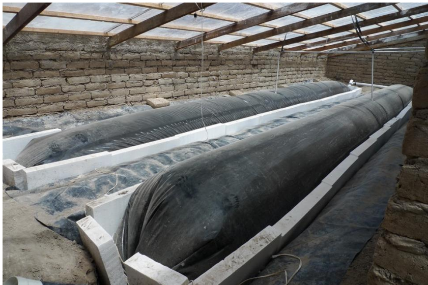
Figure 3 A. Implementation of rigid tank design in a high elevation location (Las Rocas Refuge 5130 masl). B. Tubular digester design including an insulated trench and greenhouse. Images borrowed from Dr. Jaime Martí-Herrero.
