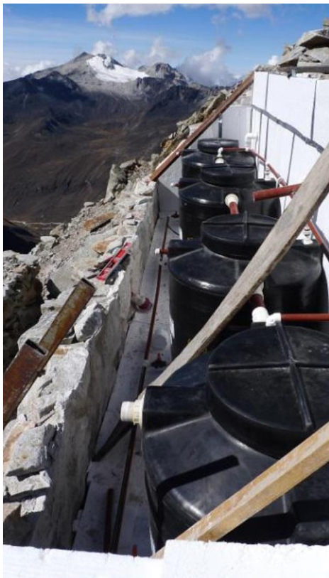
Figure 3 A. Implementation of rigid tank design in a high elevation location (Las Rocas Refuge 5130 masl). B. Tubular digester design including an insulated trench and greenhouse. Images borrowed from Dr. Jaime Martí-Herrero.
