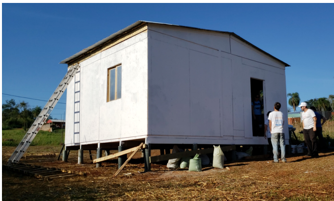
Figure 9. TECHO has constructed more than 200 housing units combining three strategies of the circular economy: modular design, wood as bio-based material, and addition of plastic components. Source: authors.
