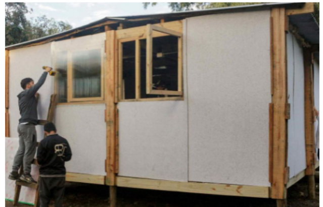
Figure 9. TECHO has constructed more than 200 housing units combining three strategies of the circular economy: modular design, wood as bio-based material, and addition of plastic components. Source: authors.
