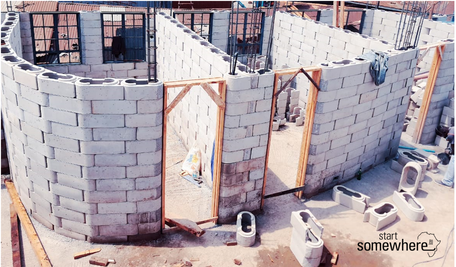
Figure 8. A structure inside the Kibera slum built with dry-stacked twist-blocks. (Source: startsomewhere.eu ).
