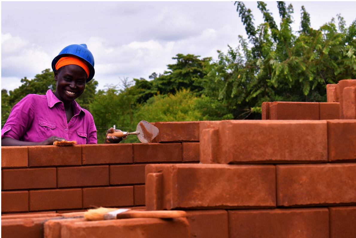
Figure 10. Interlocking stabilised soil blocks bring dry stacked into a masonry wall. (Source: hytuganda.com ).
