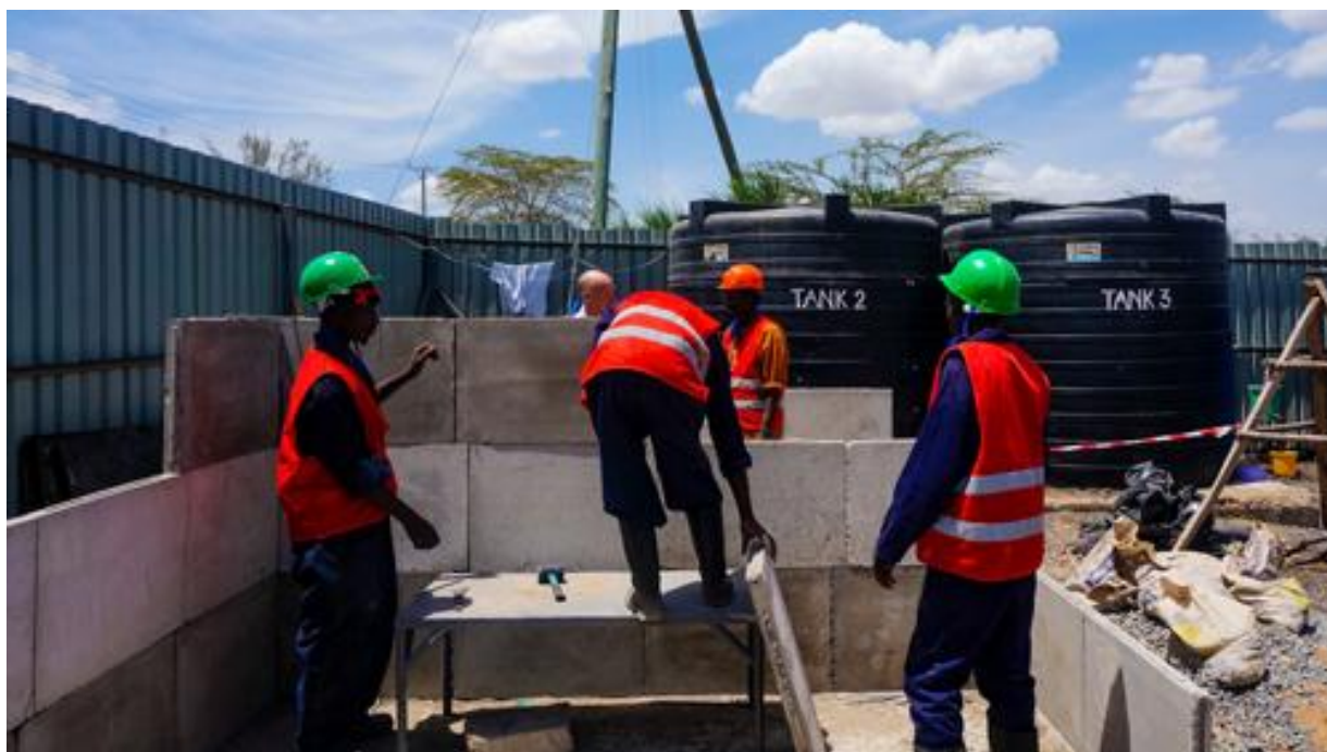
Figure 7. Kwangu Kwako team installing precast concrete panels. (Source: kwangukwako.com)
