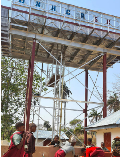
School children using a solar powered water point rehabilitated by UNHCR in Adagom community, Ogoja, Cross River State.
