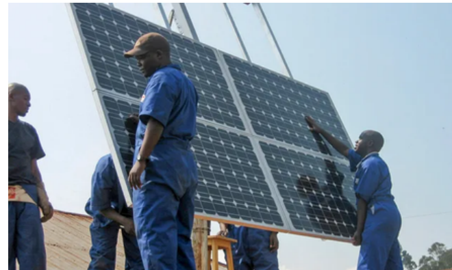
Solar panel installation
